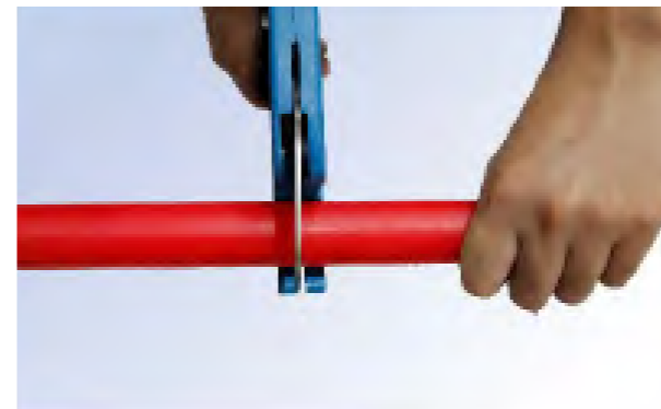
Step 1: Pipe cutting Cut the pipe vertically by RIIFO pipe cutter. Make sure to cut it quickly and precisely.
