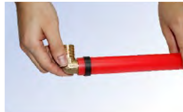
Later, insert the fitting body into the pex pipe until the shoulder of the fitting reach the pex pipe, make sure the insert is completely inside the pipe, and the contact between fitting and pipe is clean and free of impurity.
